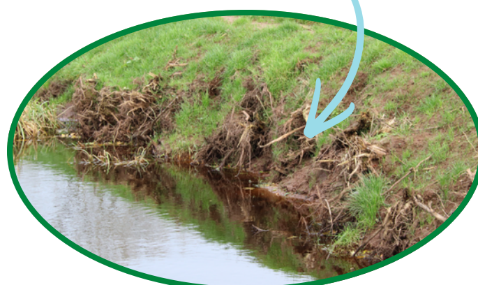
Locally sourced root wads catch silt travelling from upstream.
